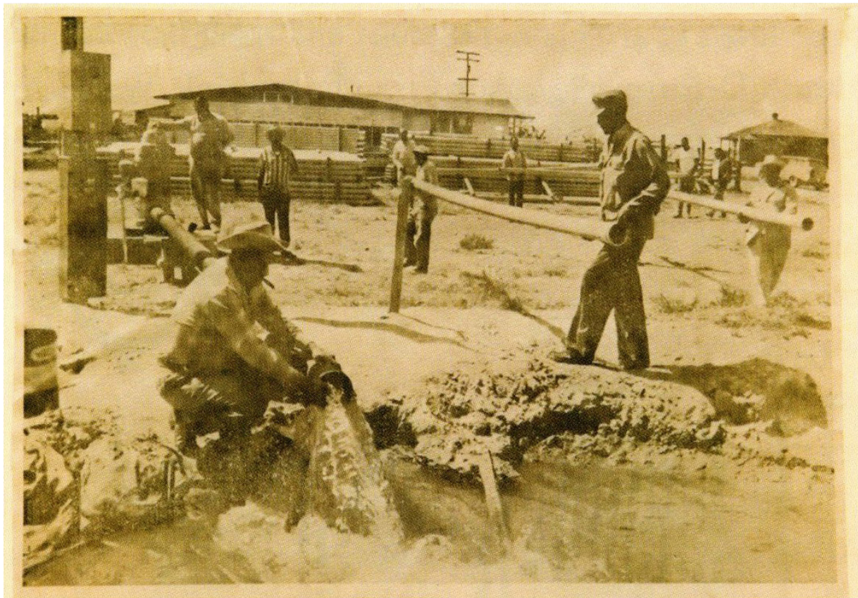
Water flows from a new 1300-foot deep well in Allensworth. Grants paid for materials, and residents laid five miles of pipe from the well to their homes. For sixty-six years the town's water has been arsenic-tainted. 1968
